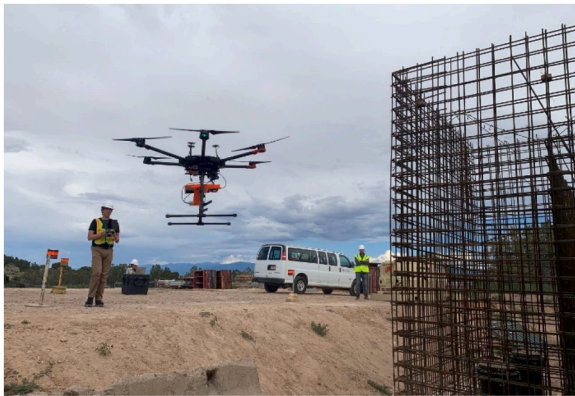
Fig. 15. UAS-RGBD data collection at the construction site, White Rock, New Mexico.
